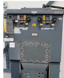
DSS B Long & Crawford T4GF3 Oil RMU
