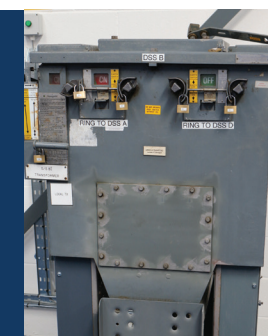
DSS B Long & Crawford T4GF3 Oil RMU
