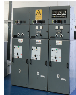
ISS GEC Alstom HWXA VCB's
