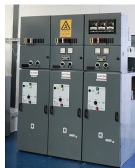
ISS GEC Alstom HWXA VCB's
