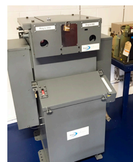
SS 4 Lucy FRMU MK2a Oil Filled RMU
