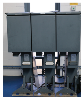
DSS A Merlin Gerin Ringmaster CE2 200A SF 6 CB 2 x SE6 630A SF 6 Switches
