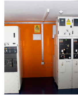
ISS Merlin Gerin Genie EVO, 2 x Merlin Gerin Genie CB6 Circuit Breaker
